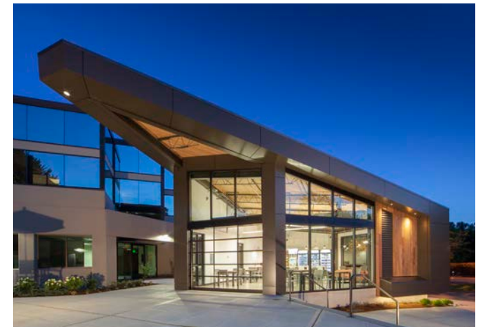
BEL-KIRK OFFICE CENTER HUB Project Size: 879 square feet 2015 | Bellevue, WA
