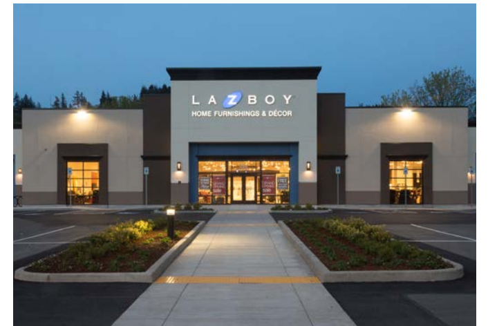
LA Z BOY EXTERIOR RENOVATION
