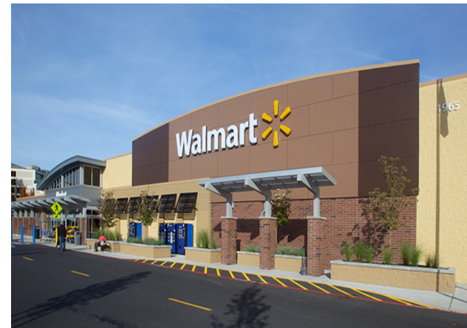
WALMART Project Size: 155,000 square feet 2013 | Tacoma, WA
