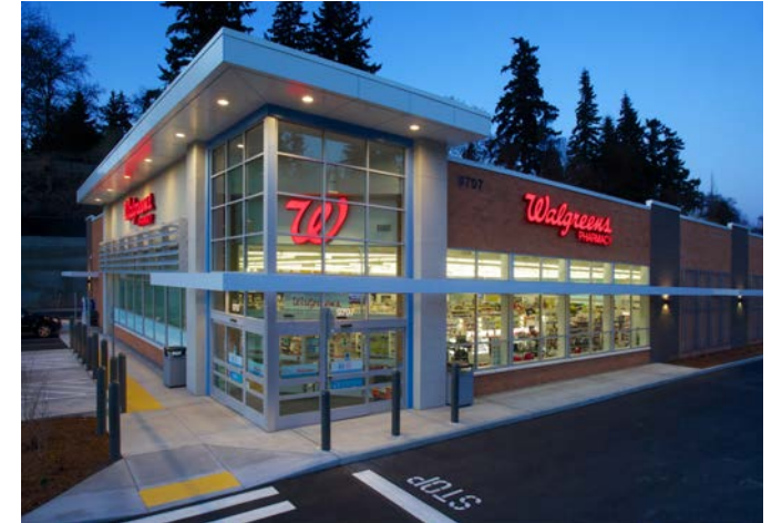
WALGREENS Project Size: 14,409 square feet 2013 | Edmonds, WA
