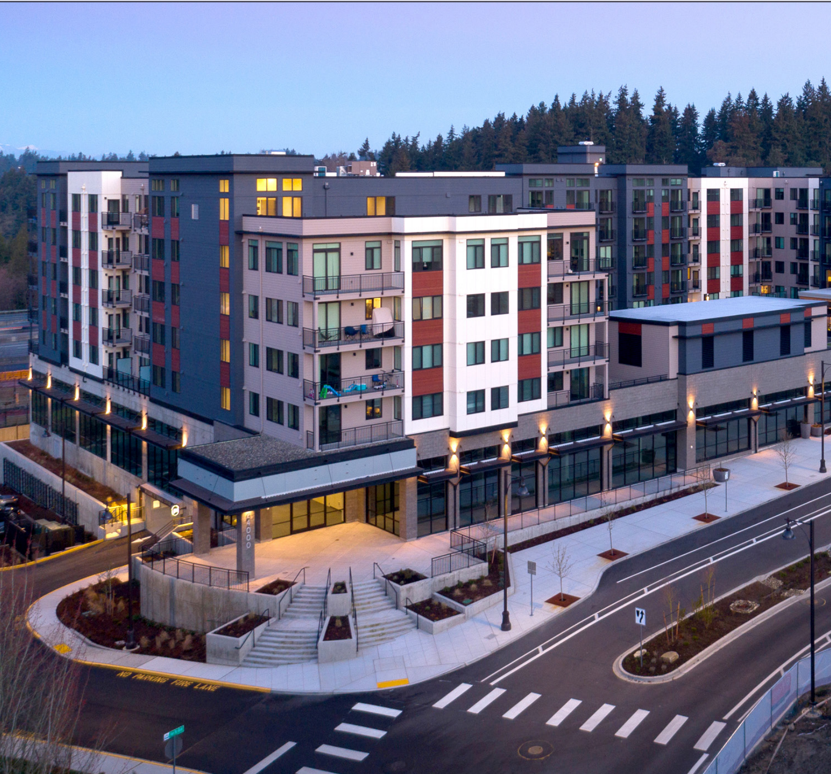
TERRACE STATION, BUILDING 1
