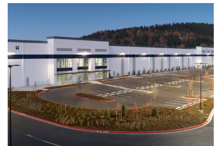
SEAPORT LOGISTICS, BUILDING 2
