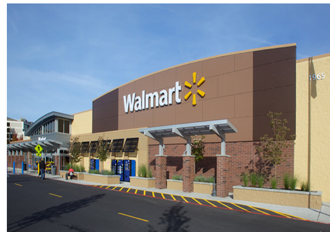
WALMART Project Size: 155,000 square feet 2013 | Tacoma, WA
