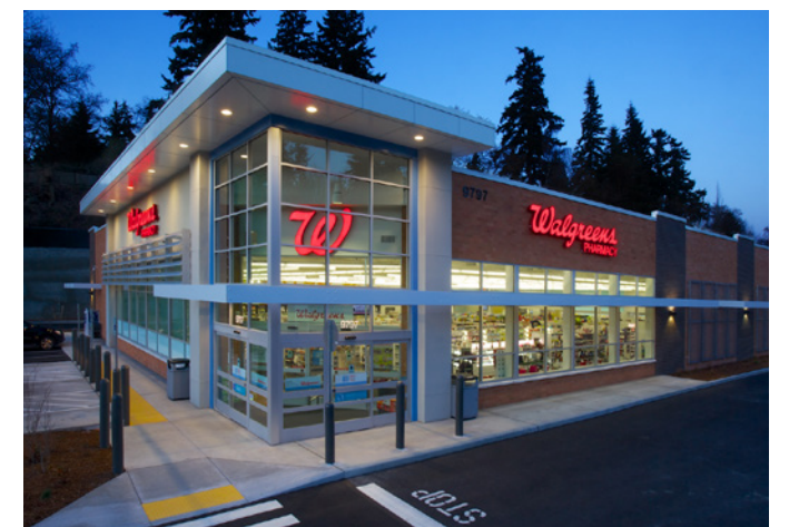
WALGREENS Project Size: 14,409 square feet 2013 | Edmonds, WA
