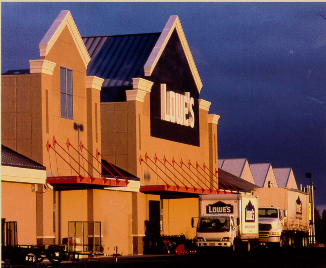
Lowe's Home Improvement Warehouse Bend, Oregon Owner: Lowe's HIW, Inc. Architect: SSOE, Inc.
