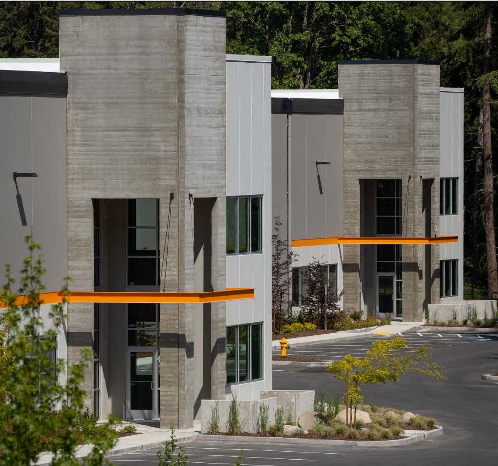
SEAWAY WEST Project Size: 64,000 - 122,000 square feet 2016 | Everett, WA
