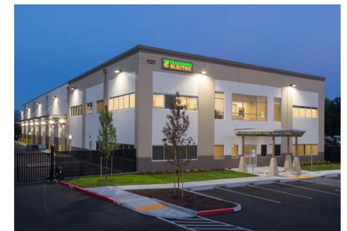
TRADESMEN ELECTRIC Project Size: 20,000 square feet 2018 | Battle Ground, WA
