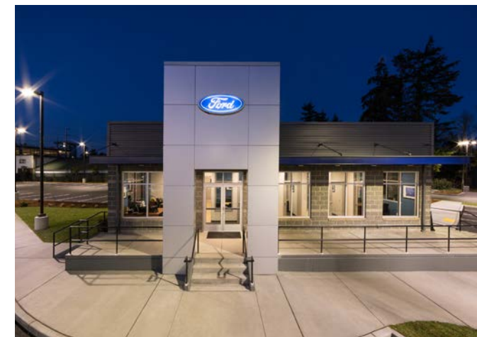
LAKWOOD FORD EXPANSION Project Size: 1,350 square feet 2017 | Lakewood, WA
