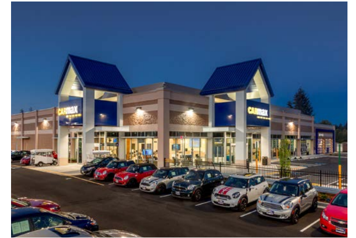
CARMAX STORE NO 7250 Project Size: 19,277 square feet 2017 | Lynnwood, WA
