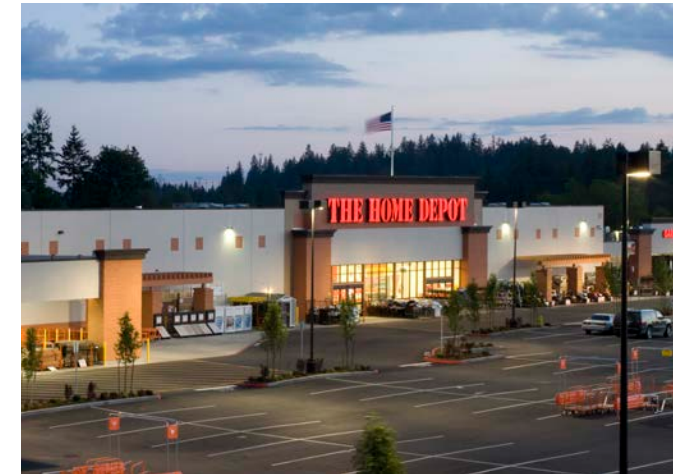
THE HOME DEPOT Project Size: 100,000 square feet 2008 | Snohomish, WA
