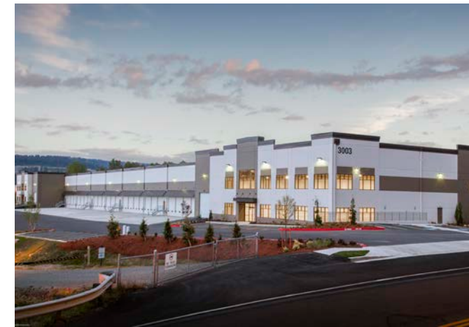
SUMNER WEST Project Size: 117,000 square feet 2016 | Sumner, WA
